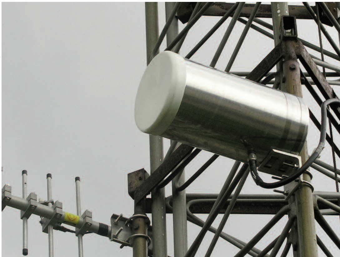
The Can Antenna mounts easily on a tower leg and takes very little space.
