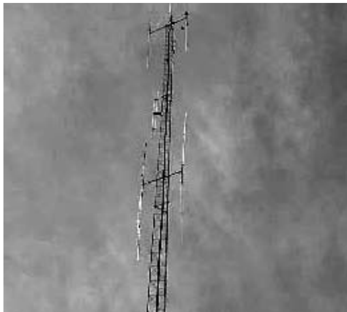
(1) Two 70 cm rib cages back to back on top left with Comet 23 cm vertical hanging down on right. Spare rib cage at midlevel on left side also mounted hanging down and currently used for UHF control. Dual band vertical used for 144.34 ATV receive and by the club station's 440 FM rig located at midlevel above spare rib cage. Other antennas used for FM repeaters and Red Cross communications. Tower is 100' high base at 750' msl elevation. (Nearby Lake Michigan is 570' msl and the 70 cm antennas favor that direction slightly, being on the west side of the tower.)
