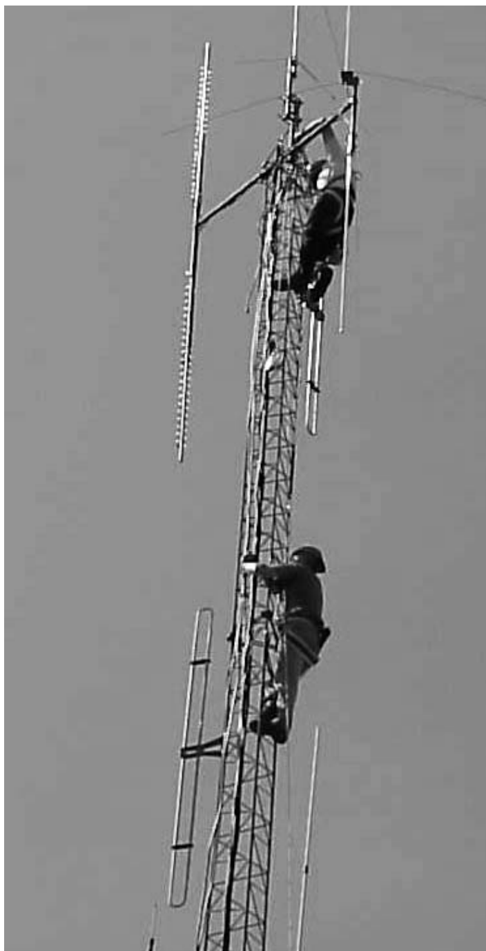
(3) Ron, K8DMR, and Dave, KF8QL (on top), installing 1/2" hard line on ATV transmit (downward pointing rub cage) on August 3rd. The receive rib cage (upper rib cage) already employed hard line but the transmit antenna had been getting by with 9913 since it was originally put up. A run of 1/2" hard line was also connected to the club's tri-band Comet in the center replacing the 9913 used there as well. The 23 cm vertical is right behind Dave at the top.
